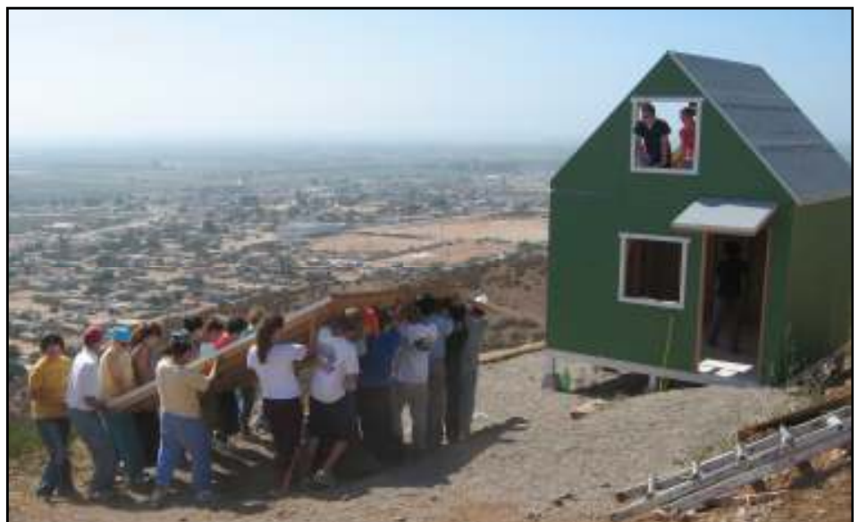
Students working together to complete the roof of the house
